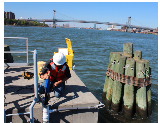
YSI EXO2 multi-parameter water quality instrument being installed by a YSI field technician at a monitoring site in New York.
